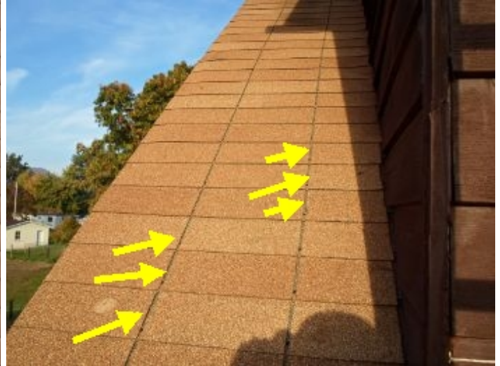
Shingles on rear of home are installed improperly and will eventually leak. They are not staggered as recommended by the manufacturer.
