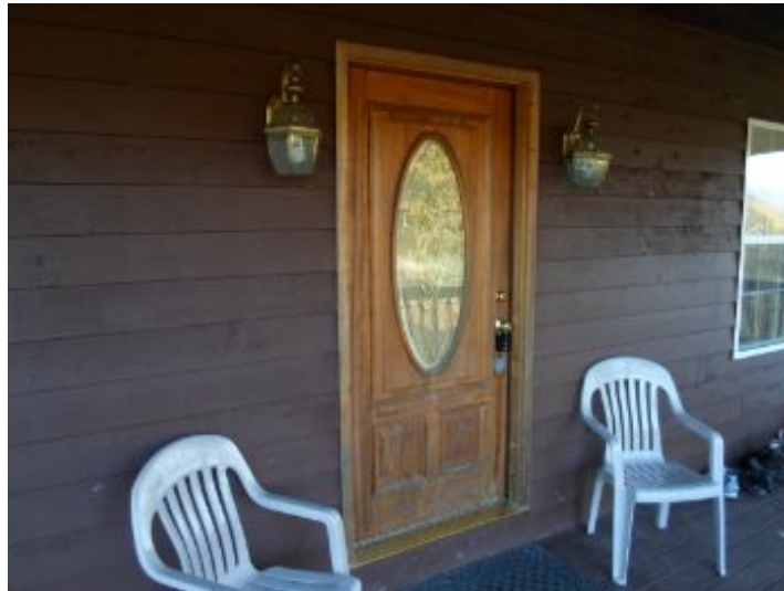
Appear in functional and in satisfactory condition, at time of inspection.
