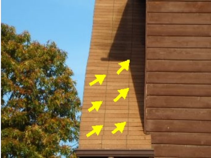
Shingles on rear of home are installed improperly and will eventually leak. They are not staggered as recommended by the manufacturer.
