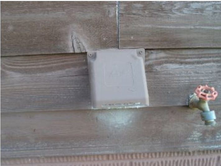
Appeared functional at time of inspection
