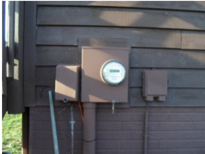
Appeared functional and serviceable, at time of inspection.
