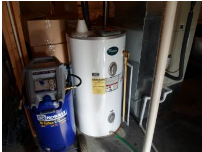
Appears to be in satisfactory condition -- no concerns.
