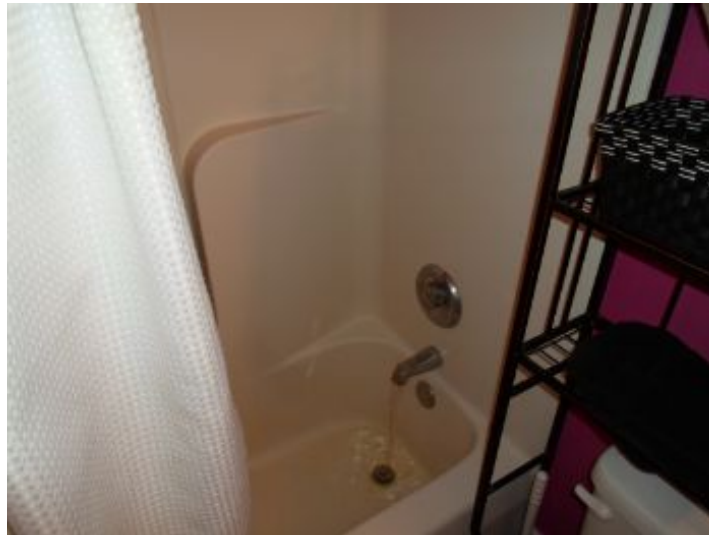
Appeared satisfactory and functional, at time of inspection.
