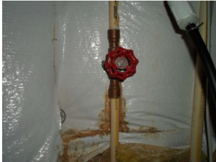
Appeared functional at time of inspection.
