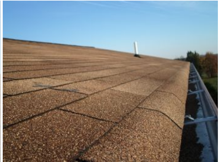
Shingles on rear of home are installed improperly and will eventually leak. They are not staggered as recommended by the manufacturer.
