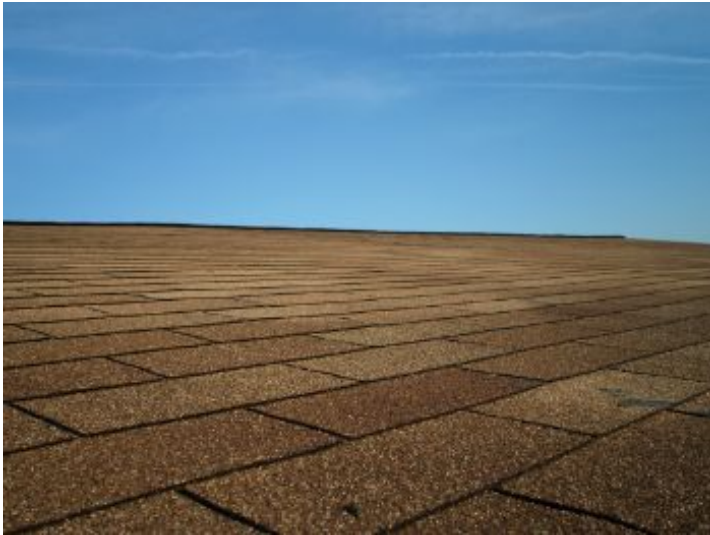
Shingles on rear of home are installed improperly and will eventually leak. They are not staggered as recommended by the manufacturer.
