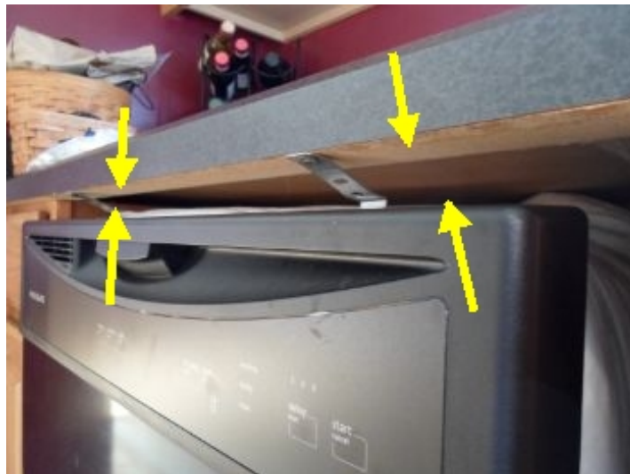
Needs to have the legs adjusted up so that there isn't such a big gap from the counter top.
